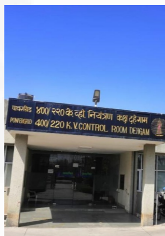
Powergrid Co. Of India
